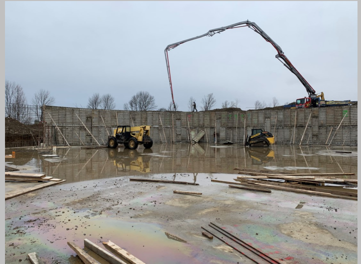
Concrete walls poured in succession by a pump truck for the 1.8 million gallon waste storage.
