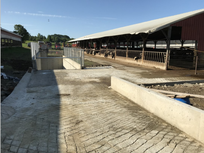
Concrete manure scraping pad and concrete reception pit to capture manure from adjacent barns.
