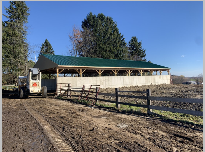
Covered pack manure storage and roof runoff management system for Wilmar Farms, in Wethersfield.
