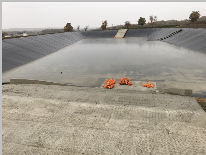
Plastic lined, 6 million gallon earthen storage completed in fall of 2019 for Baker Brook Farms.
