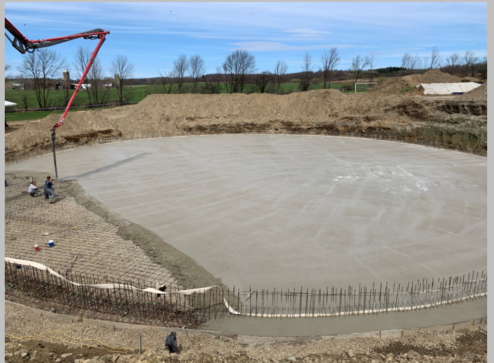
Pouring of the concrete floor for the storage tank.
