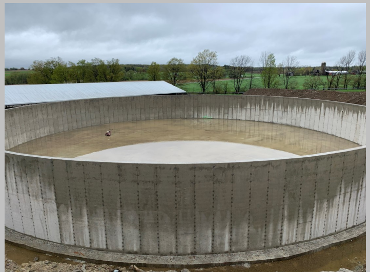
Completed 1.8 million gallon concrete waste storage tank.
