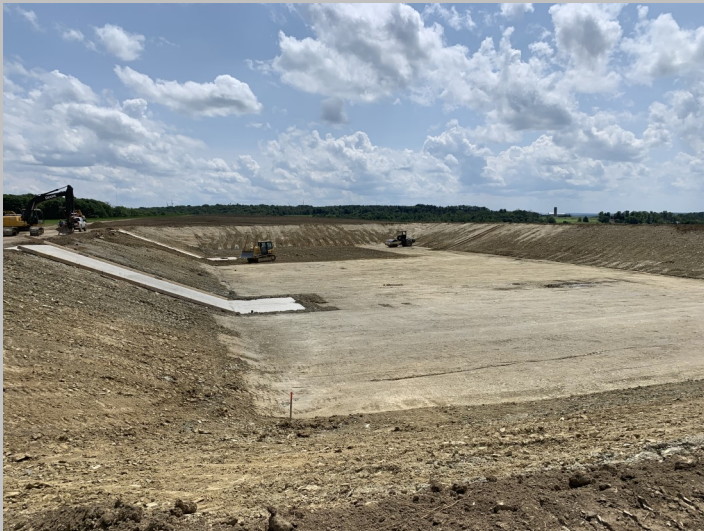
Compacted clay earthen storage with concrete pump pads at Conrad Farms in Wethersfield.
