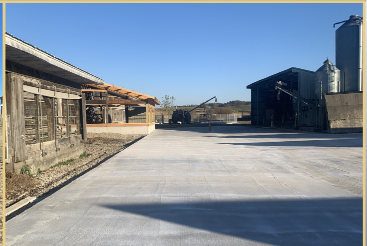
Heavy Use Area: The concrete heavy use area directs silage leachate runoff from the farms bunks into the nearby reception pit.
