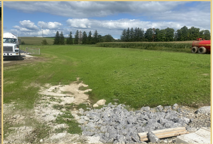
Diversion Ditch After: Post hydroseeding, the conservation mix has established on the erosion fabric.
