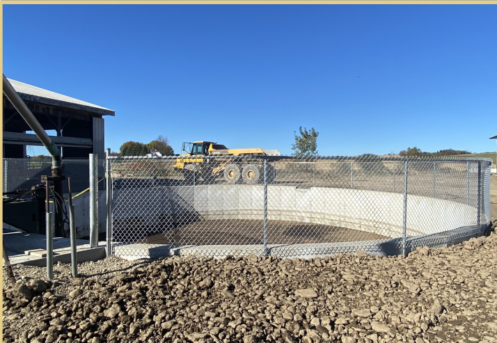
Reception Pit: This reception pit provides additional storage during winter months, and can be pumped to the main storage, or pumped out and spread.
