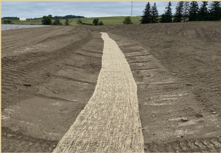
Diversion Ditch Before: This depicts the construction of a diversion ditch with erosion fabric.
