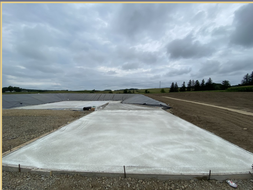
Concrete Ramp: This ramp will allow the farm to clean out solids from the bottom of the manure storage. Maintenance is key to BMP's remaining useful and effective.
