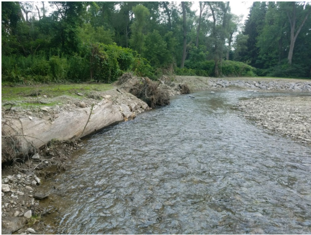
Log revetments are placed and cabled in to armor the streambank.
