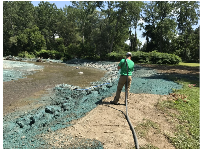
All exposed soil was hydro seeded in hopes that the roots would further stabilize the bank.
