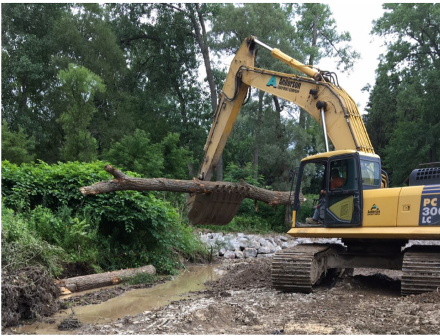
Debris was removed and used as revetments.
