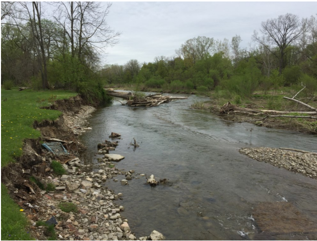
Fast moving water has scoured the stream bank undermining trees and taking away land.
