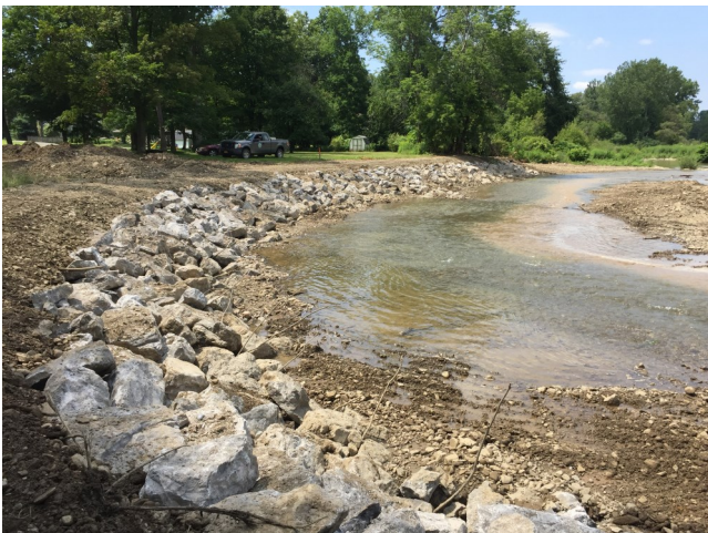
Large rock was installed along the bend, the rock was toed in so that it is more resistant to being undermined by the flow.
