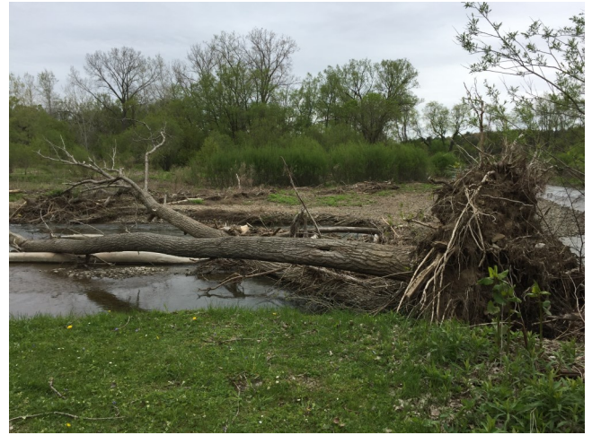
Large woody debris filled the streambed and caused further backups and erosion.
