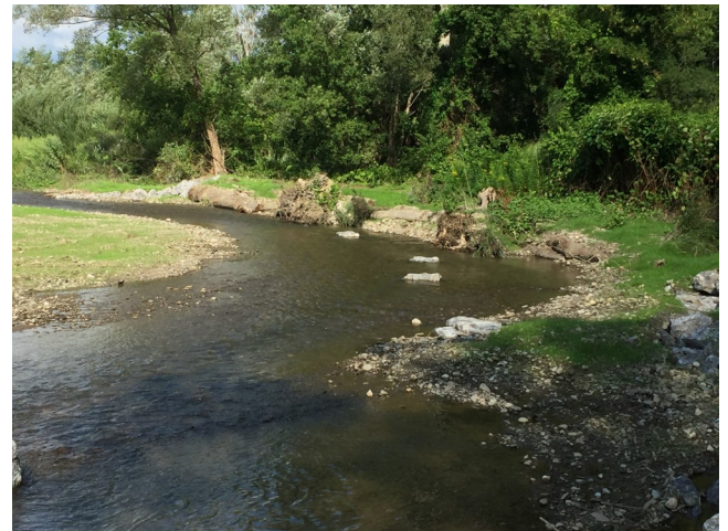
With log revetments, rock vanes, and bank armoring installed, the flow is deflected off of the soil and reduces erosion.
