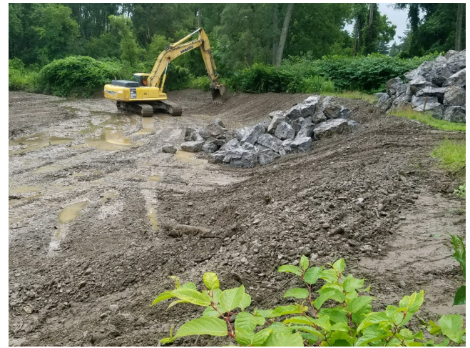
The stream flow was diverted to allow the excavator to reshape the bank of the channel.
