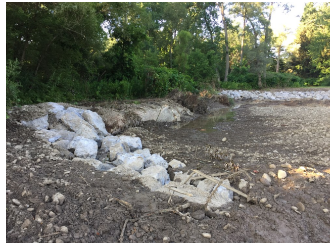
Rock veins were installed to deflect water away from the streambank.
