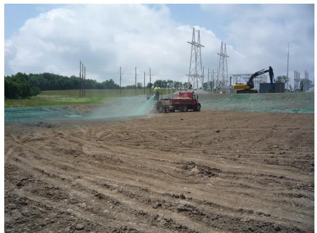
During: Wyo. Co. Highway Dept. staff operate the Finn T90 hydroseeder to cover the 2 acre area
