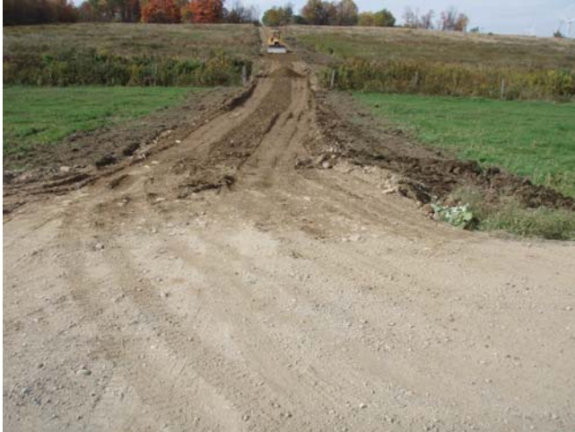
Animal Laneway under Construction
