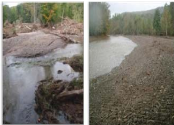
Stream in Delaware County damaged by flooding (left). Stream after ESI Program implemented (right).
