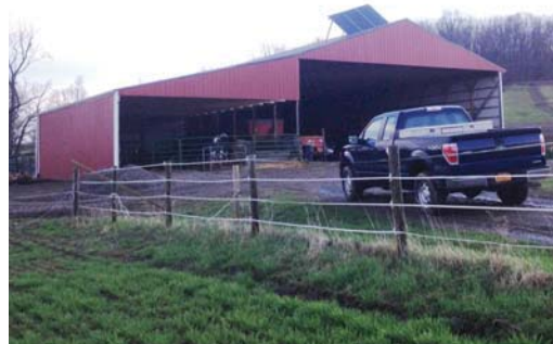
Yates SWCD installed solar panels for a grazing water system.
