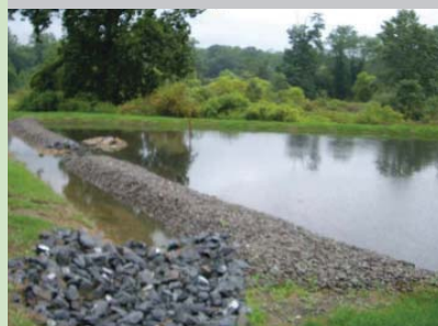
Bioretention basin at Warwick HS captures parking lot runoff (above). Basin in operation (below).
