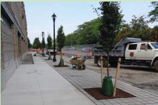
Street trees and permeable pavers in the East Village of Rochester by Monroe SWCD.
