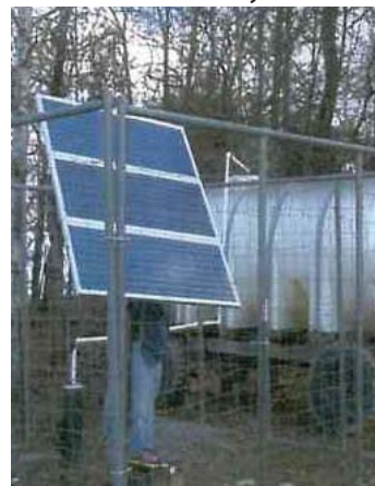
Essex SWCD installed a solar panel to pump water for cattle.
