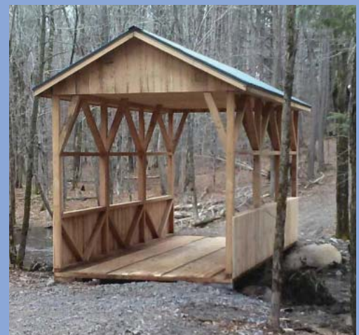
Covered bridge connecting recreational trails built by Jefferson Conservation District.
