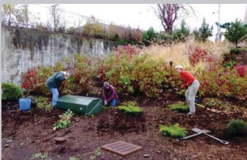
Rain garden at SUNY Orange installed by Lower Hudson Coalition of Conservation Districts.
