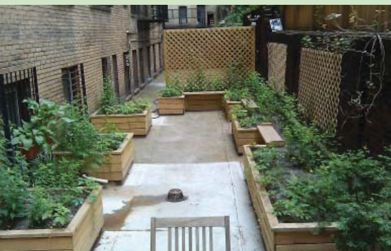
Stormwater planters installed by NYC SWCD for roof runoff capture and retention.
