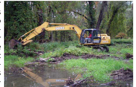
Honeoye Creek in Ontario County was remediated by the Ontario SWCD to remove obstructions and restore flow after flooding.
