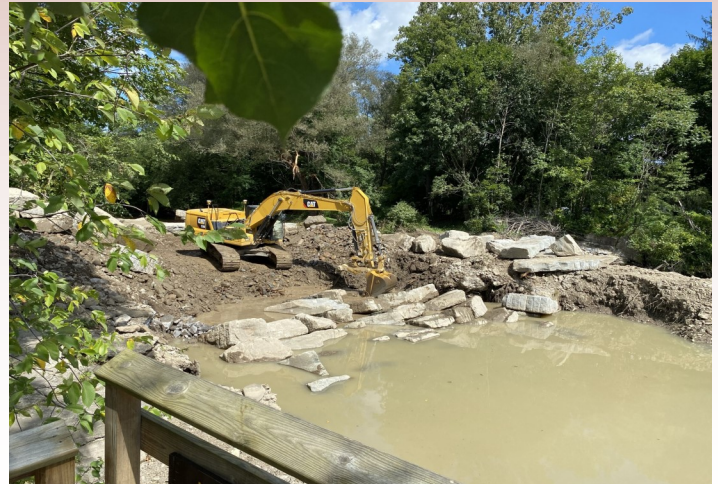
Contractor carefully placing rock to better improve fish habitat and upstream connectivity
