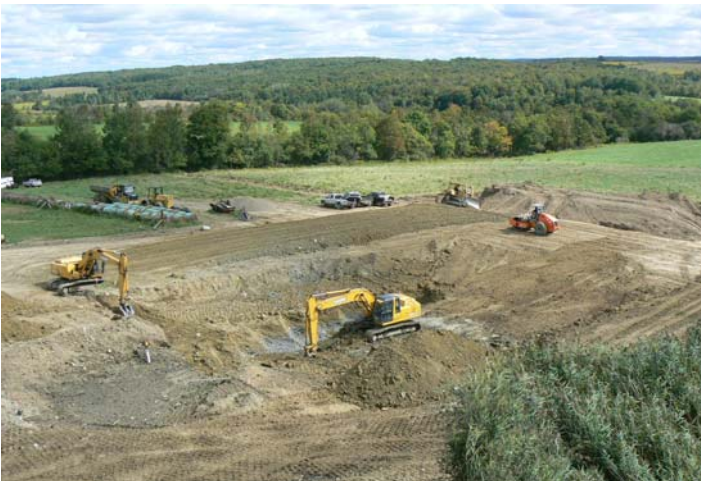
Construction of the Earthen Manure Storage
