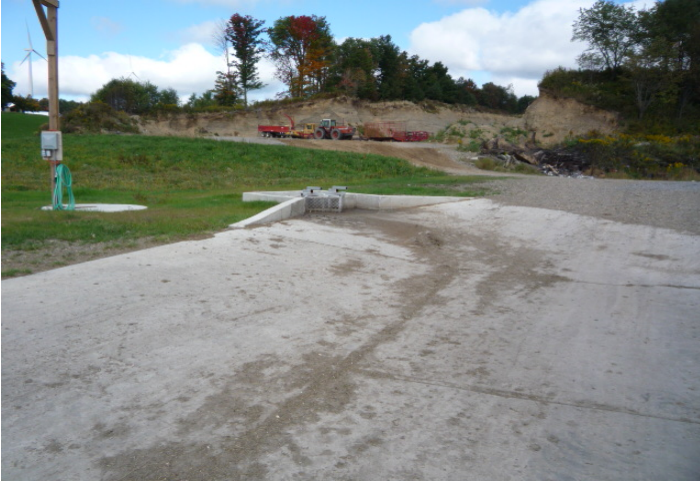
Silage Leachate Collection
