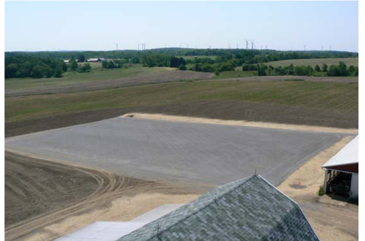
Ag bag storage pad and an integrated perimeter access road maintains traffic flow during harvest
