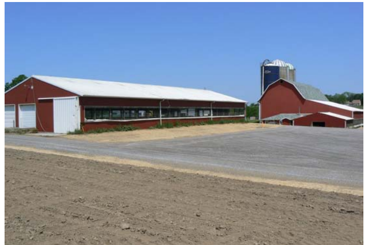
Completed Ag Bag Pad and Diversion
