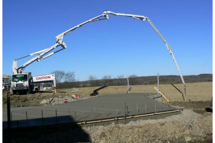
Construction of Ag Waste Transfer Area
