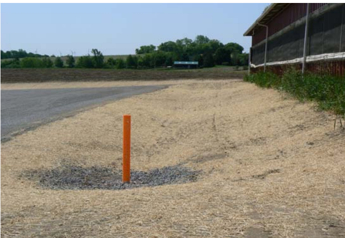
Diversion w/ surface inlet to catch and redirect roof runoff and melting snow drifts
