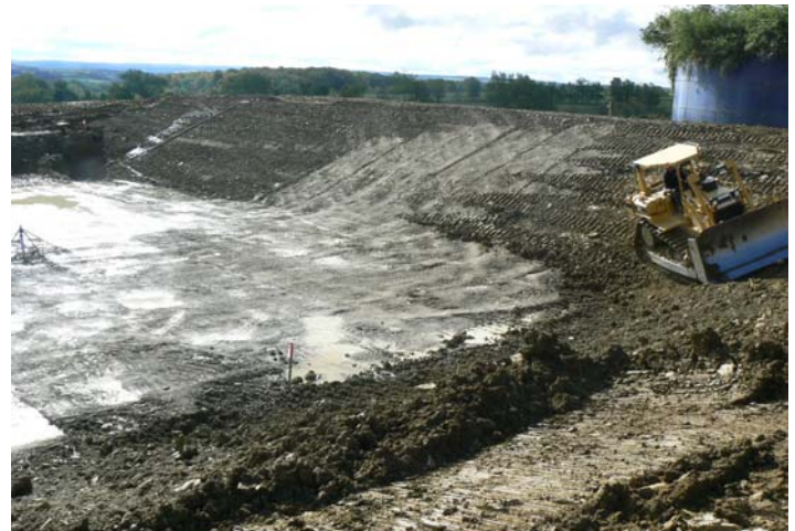
Completed Manure Storage
