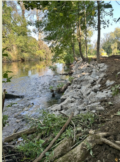
100 ft of Rock Rip-Rap Streambank Stabilization
