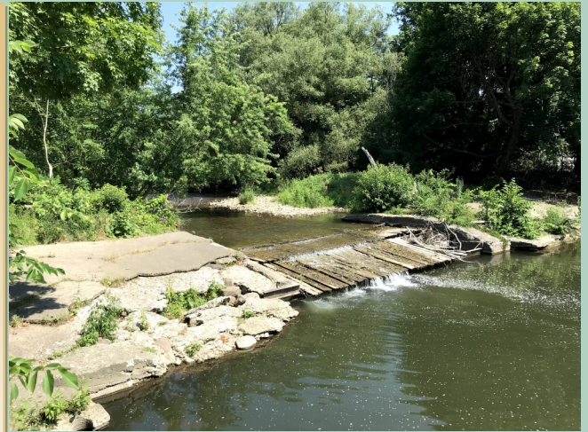
PIKE DAM REMOVAL - WYOMING COUNTY FAIRGROUNDS
