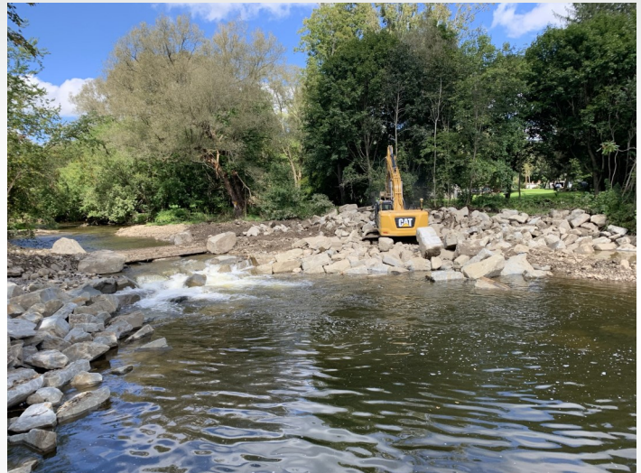
The stream channel was re-aligned while the remainder of construction is being finished, thereby restoring the pool.
