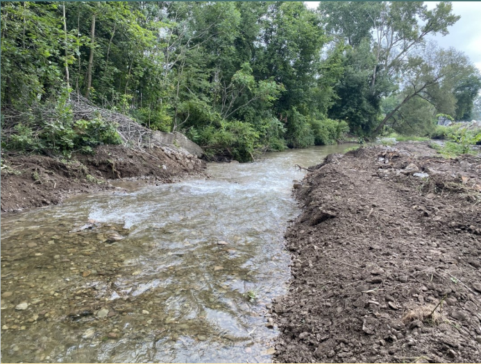
A temporary bypass channel was excavated adjacent to the dam to dewater the main stream prior to construction.
