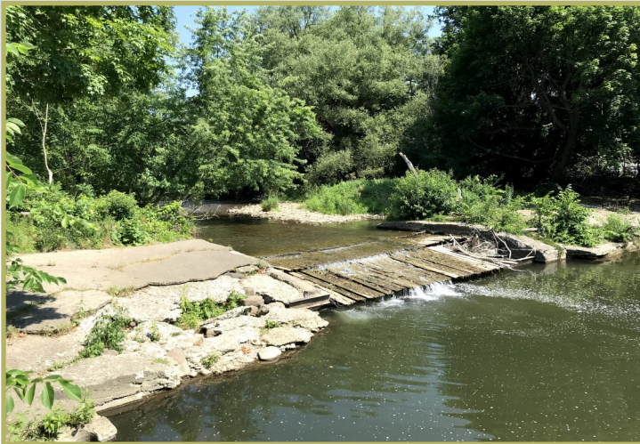
July 2020: Degradation of concrete and wooden planks is very apparent during times of low flow
