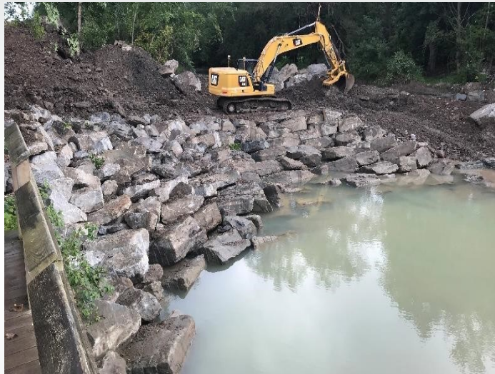
This picture depicts one side of the engineered rock riffle being completed in a staggered staircase formation.
