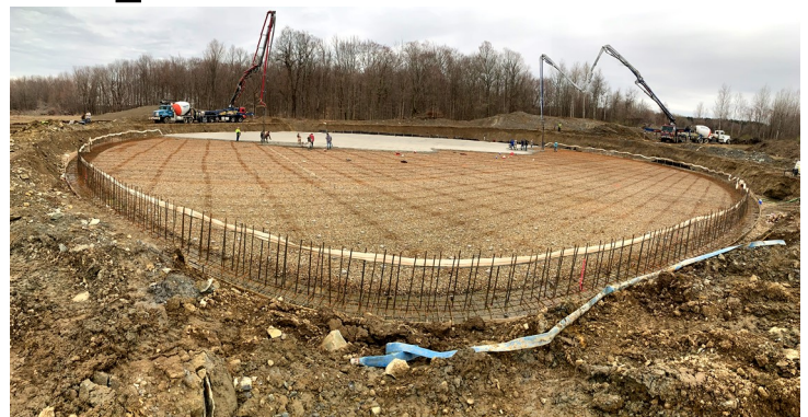
Pouring the concrete floor for the manure storage structure with the rebar, forms, and dry seal in place.
