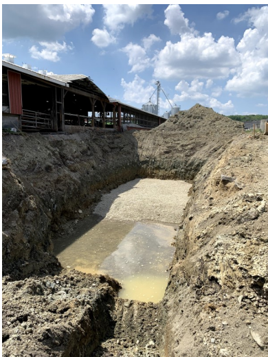
Excavation and construction for a covered reception pit and transfer line that will connect to the new storage structure.
