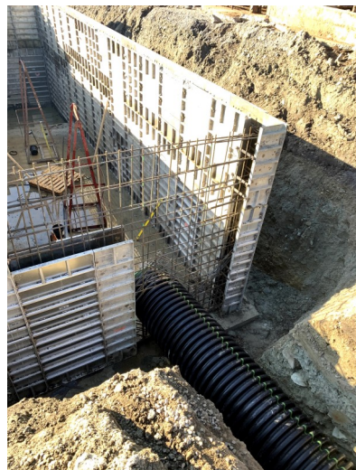
Excavation and construction for a covered reception pit and transfer line that will connect to the new storage structure.
