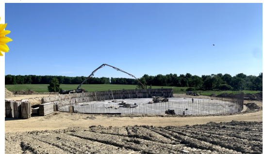
Rebar and forms set for the first section of the concrete wall pour.
