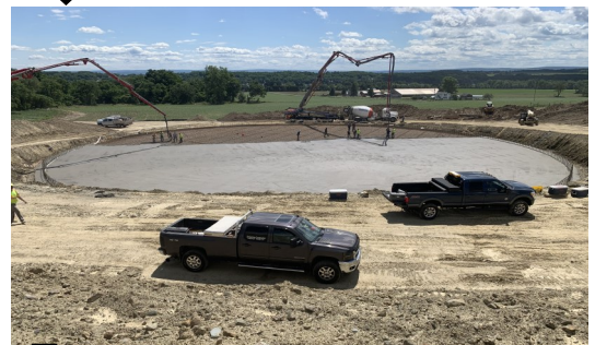
Leveled stone, rebar, forms, and dry seal in place for the concrete floor pour.
