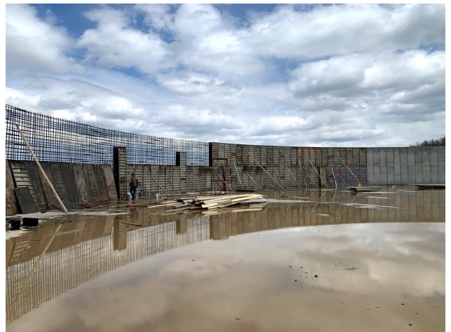
↑ First concrete wall section completed, rebar and forms going up for the second.
