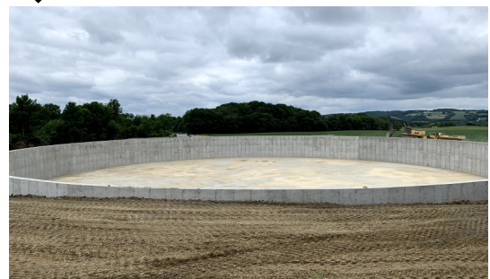
Completed and backfilled concrete manure storage structure.
