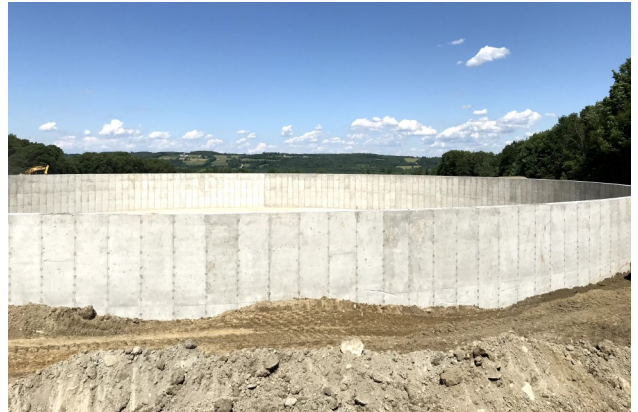
↑ Completed manure storage structure with backfilling underway.
