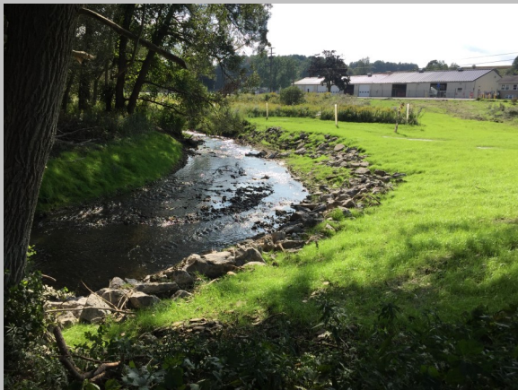
Streambank Protection at Rock Glen Baptist Church
