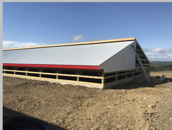
Construction of Covered Waste Storage at Deere Stone Farms, LLC
