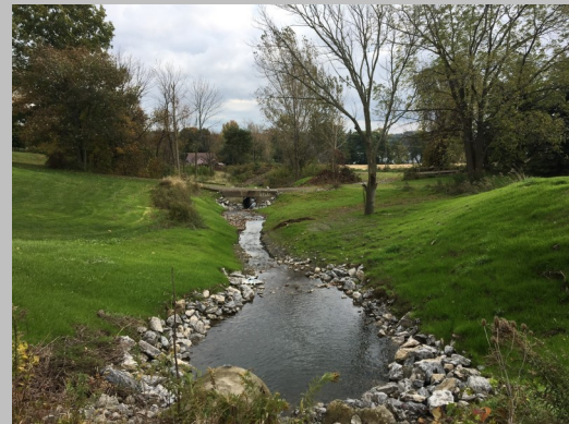
Private Dr 1, Plunge Pool and Diversion Ditch, Silver Lake
