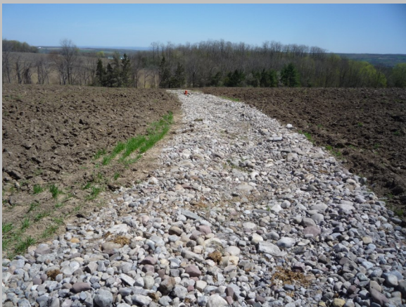
Harkins Dairy, LLC Lined Waterway with Underground Outlet
