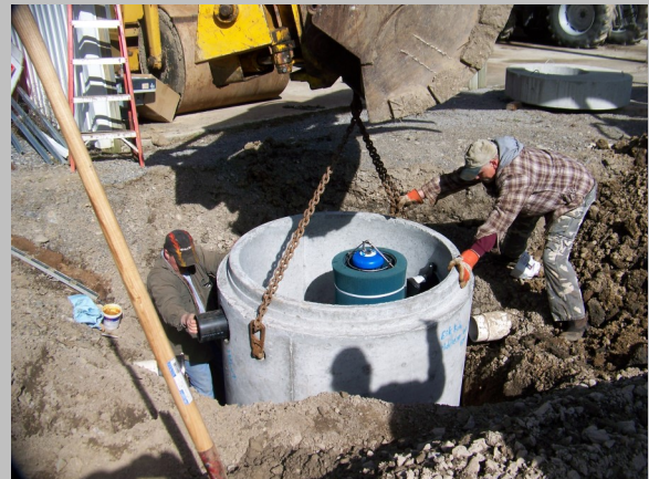
Town of Middlebury Highway Dept. Oil Separation Unit
