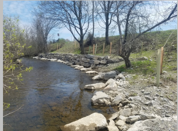
Streambank Stabilization at Shearing Rd, Gainesville
