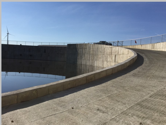
Construction of Waste Storage at Davis Valley Farm, LLC
