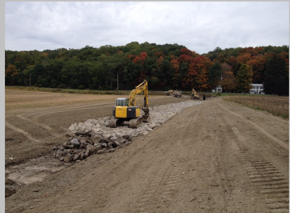
Rock-lined waterway under construction at R. L. Jeffres & Sons Farm
