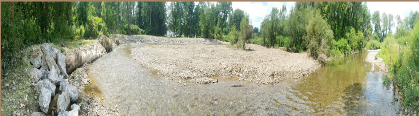
Onsite logs were used as log revetments to protect the bank on the Wiscoy Creek
