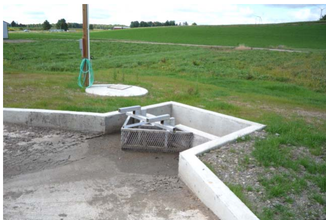
Silage Leachate Management System completed at Davis Valley Farm in the Cattaraugus Creek Watershed.
