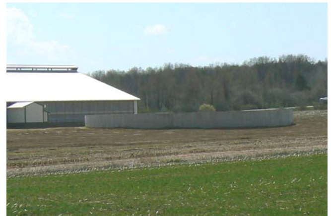
Concrete waste storage & waste transfer system completed at East Koy Valley Farms in the East Koy Creek Watershed.
