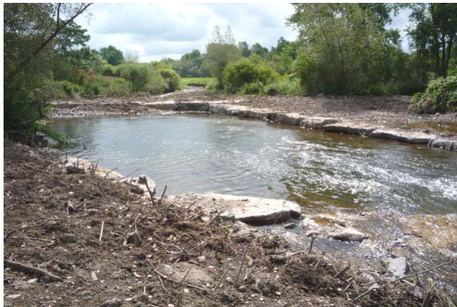
Rock rip-rap channel block to divert stream flow back to its original channel.
