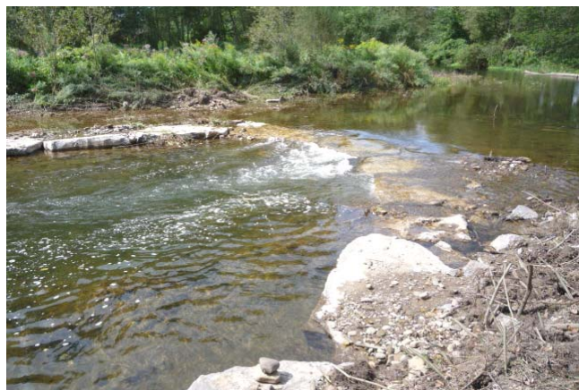
Rock grade control structure completed on the Wiscoy Creek.
