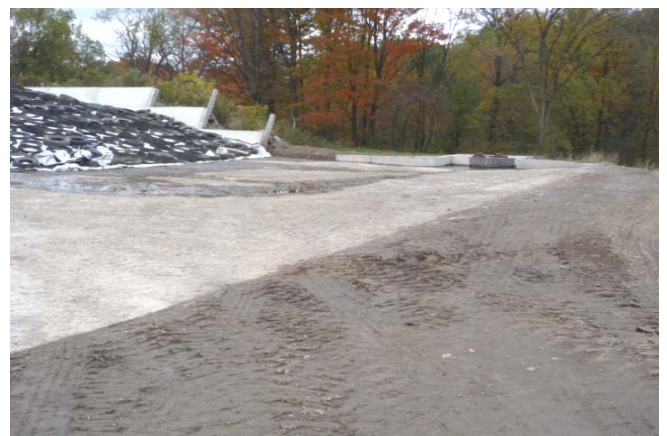
Silage Leachate Management System completed at Seewaldt Bros. Dairy Farm in the Tonawanda Creek Watershed.
