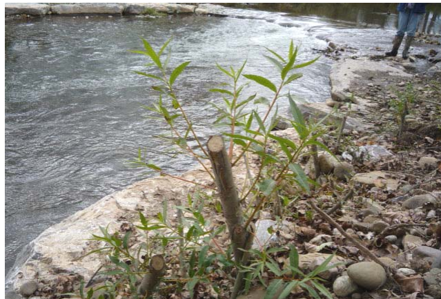
Live willow stakes established for bank stabilization along the project area.
